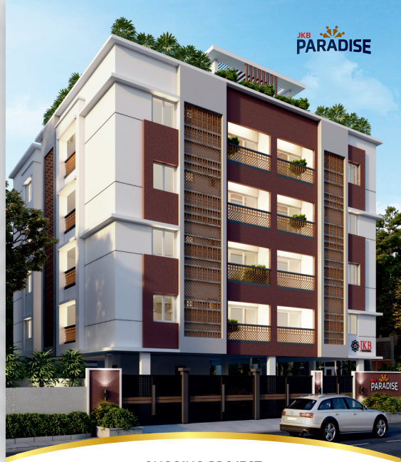
ONGOING PROJECT 📍 VALASARAVAKKAM MAJESTIC COLONY
